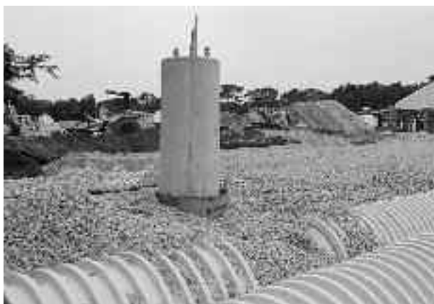
Figure 15 – Chamber bed placed around light post.
